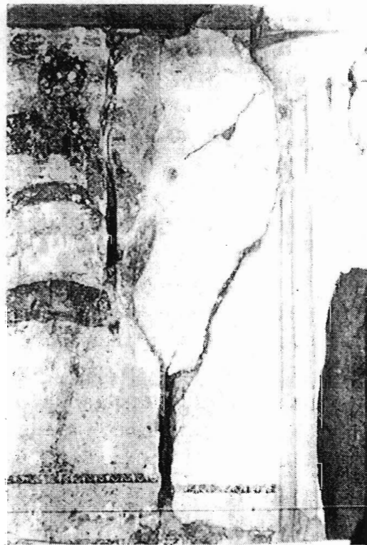
Figure 10. Krisis Tomb. The differential settlement caused failures and displacements on the front wall
